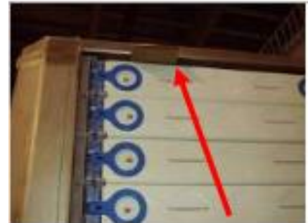
Figure 24 - Permeate pipe clips engaged on the permeate pipes
