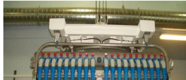
Figure 26 - Lowering cassette into membrane tank
