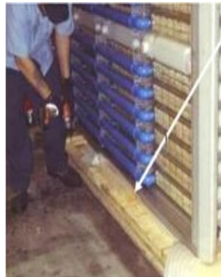
Figure 5 - Removing shipping braces (attached to base of crate)
