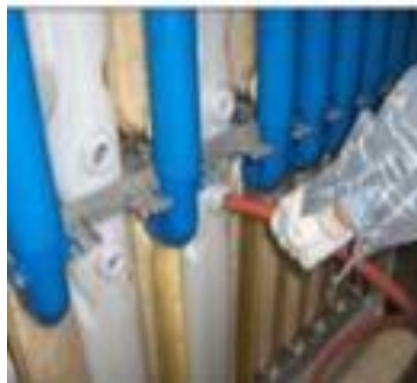
Figure 22 - Filling blank modules
