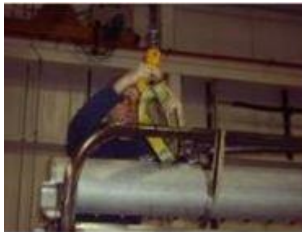
Figure 15 - Disengaging hoist & sling
