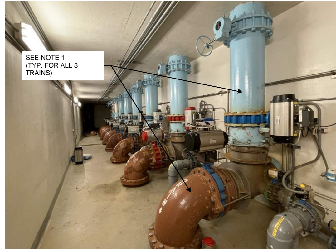
2 MEMBRANE DRAIN PIPE GALLERY 001-PK-001 NTS
