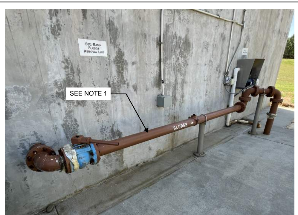
1 SED. BASIN SLUDGE REMOVAL NTS
