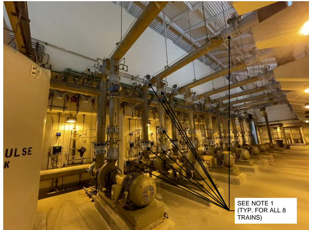
1 MEMBRANE PERMEATE PUMP GALLERY 001-PK-001 NTS
